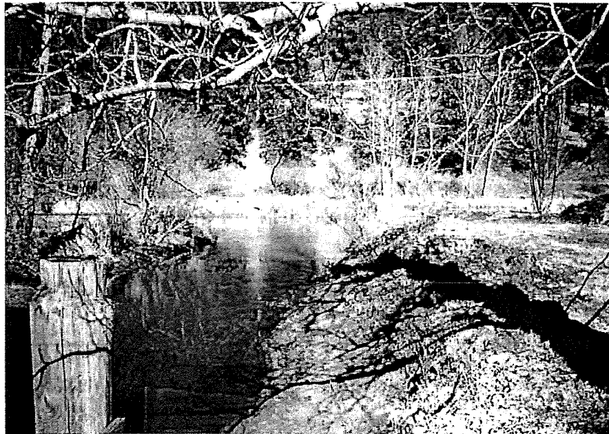
ENTRANCE TO BASIN. WAS DEEPEMED & DEVEGETATED. NO EVIDENCE OF TURBIDITY CONTAINMENT.
