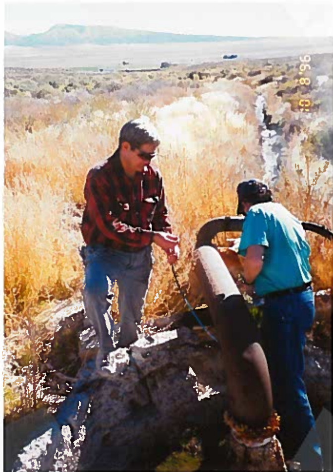
CLELLAND & FARLEY INSTALL GPS TAG TO WELL HEAD.
