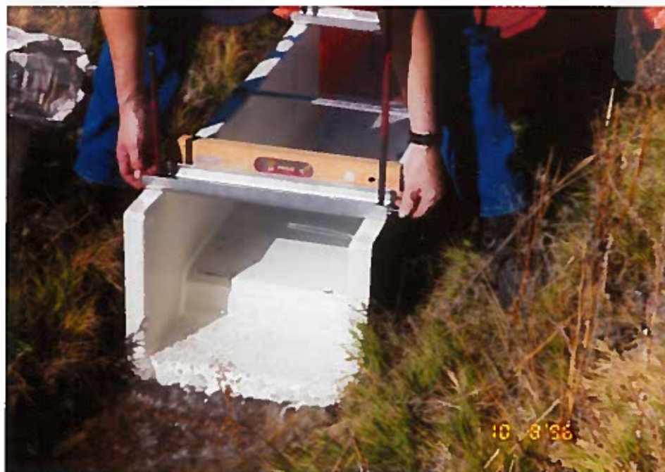
SETTING WEIR IN DITCH.
