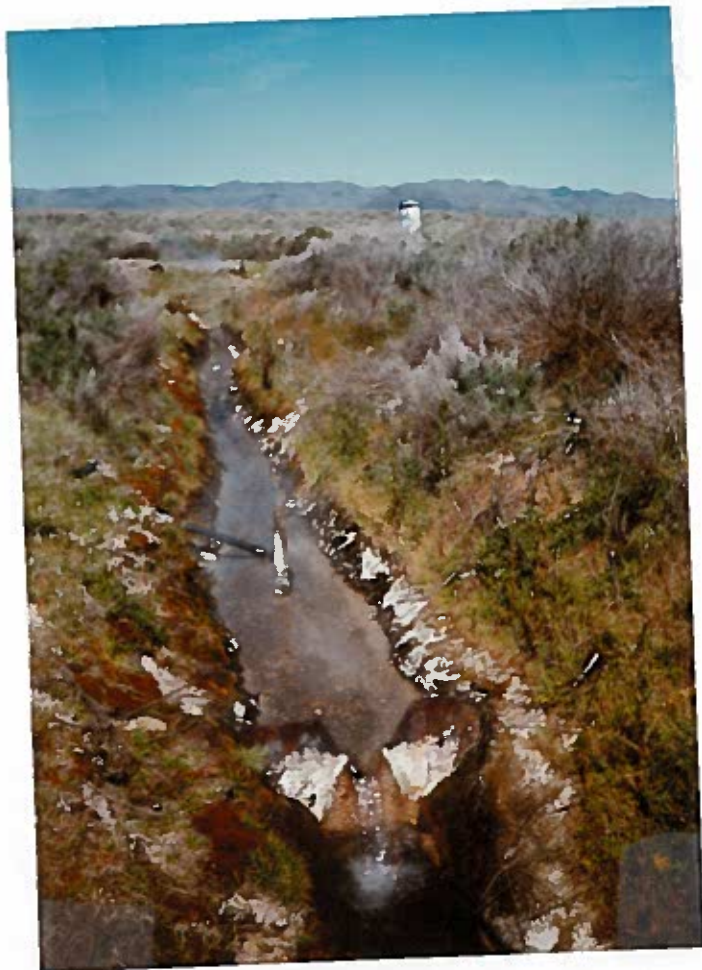
V-NOTCH WEIR NEEDS IMPROVEMENTS TO BE ACCURATE.
