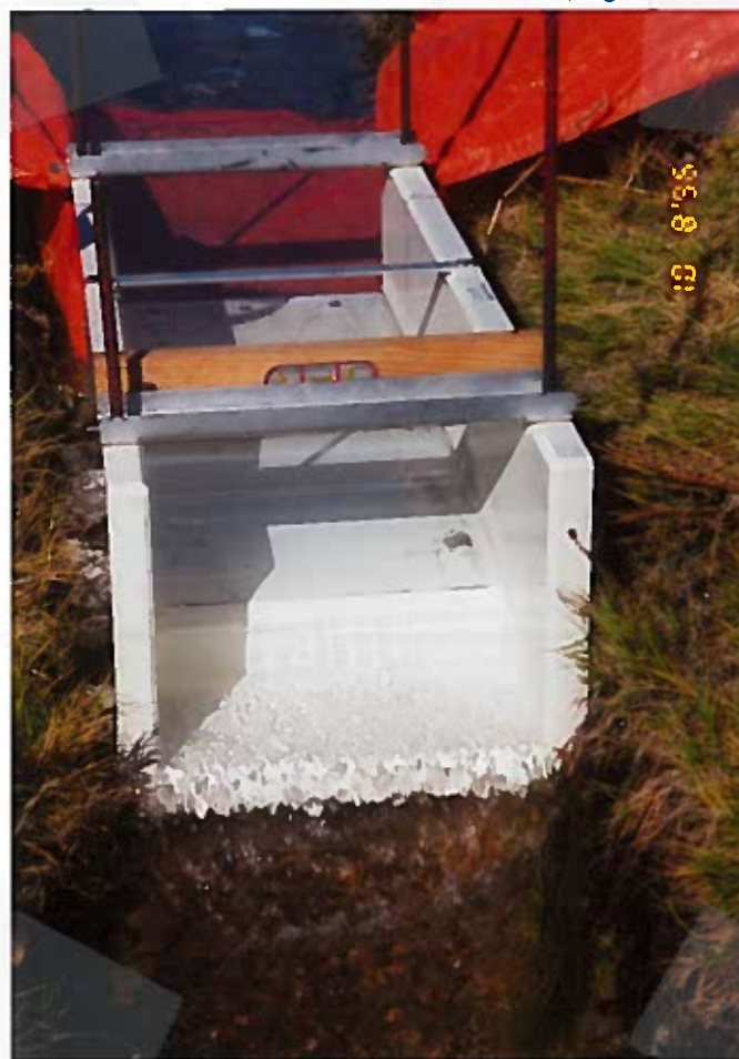
FINAL SET-UP OF WEIR IN HOT WELL DITCH TO FARLEYS.
