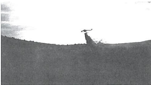
Helicopter Hydroseeding Bunker Hill Hillsides, Fall 1998.
