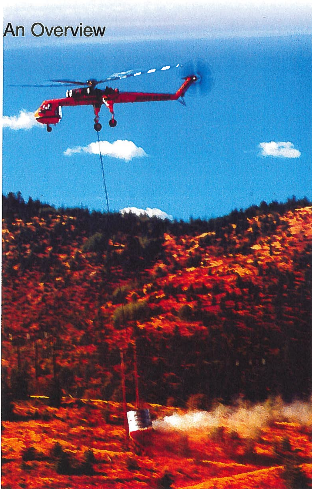
Aerial Hydroseeding of Bunker Hill Hillsides, September 1998
