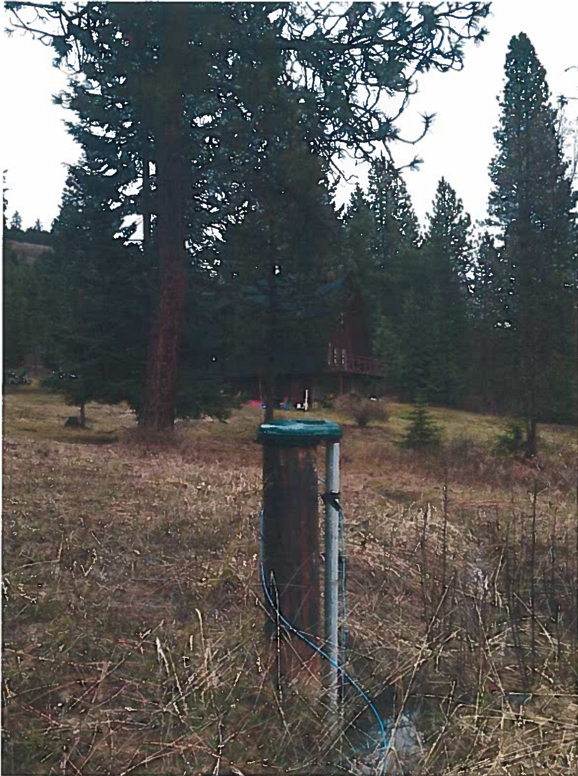
4) Point of Diversion – Replacement Well
