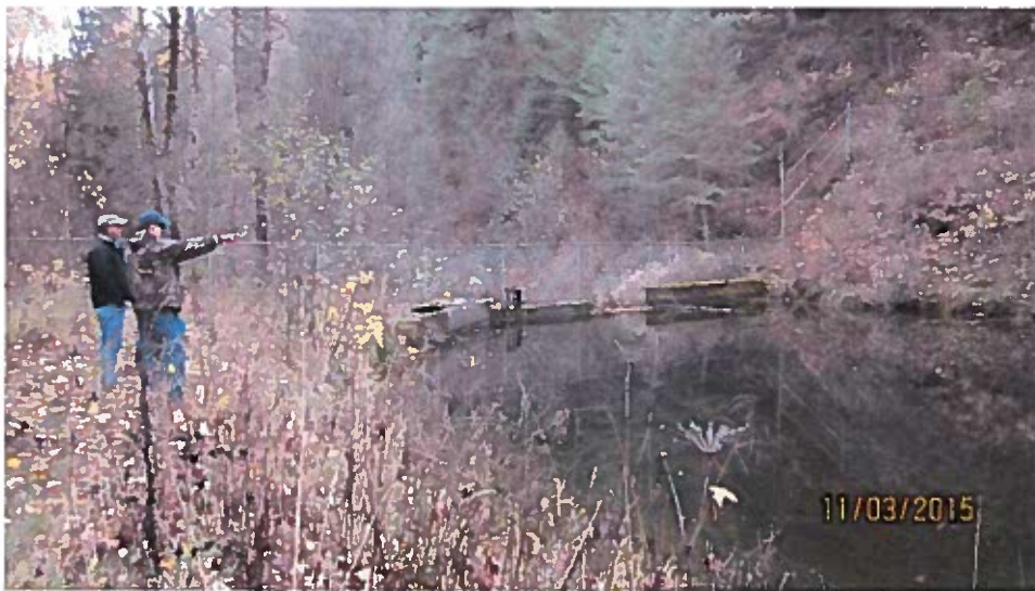
LOOKING SOUTH AT DAM AT HEADGATE, EMERGENCY SPILLWAY & PIPELINE VAULT
