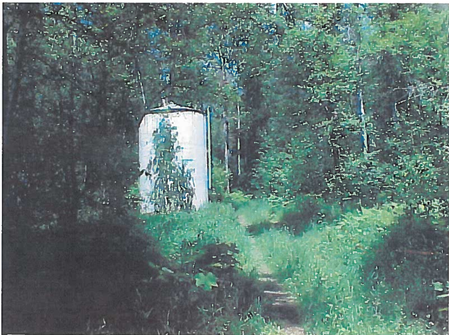
OLD STORAGE TANK
