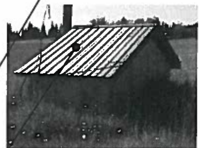
Existing well hand dug well
