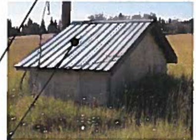
Existing well hand dug well
