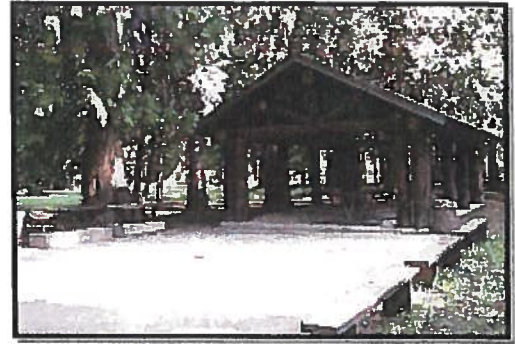
Picnic pavilion with slab extension.
