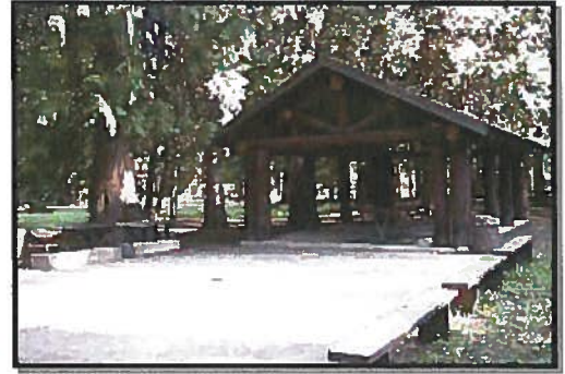
Picnic pavilion with slab extension.
