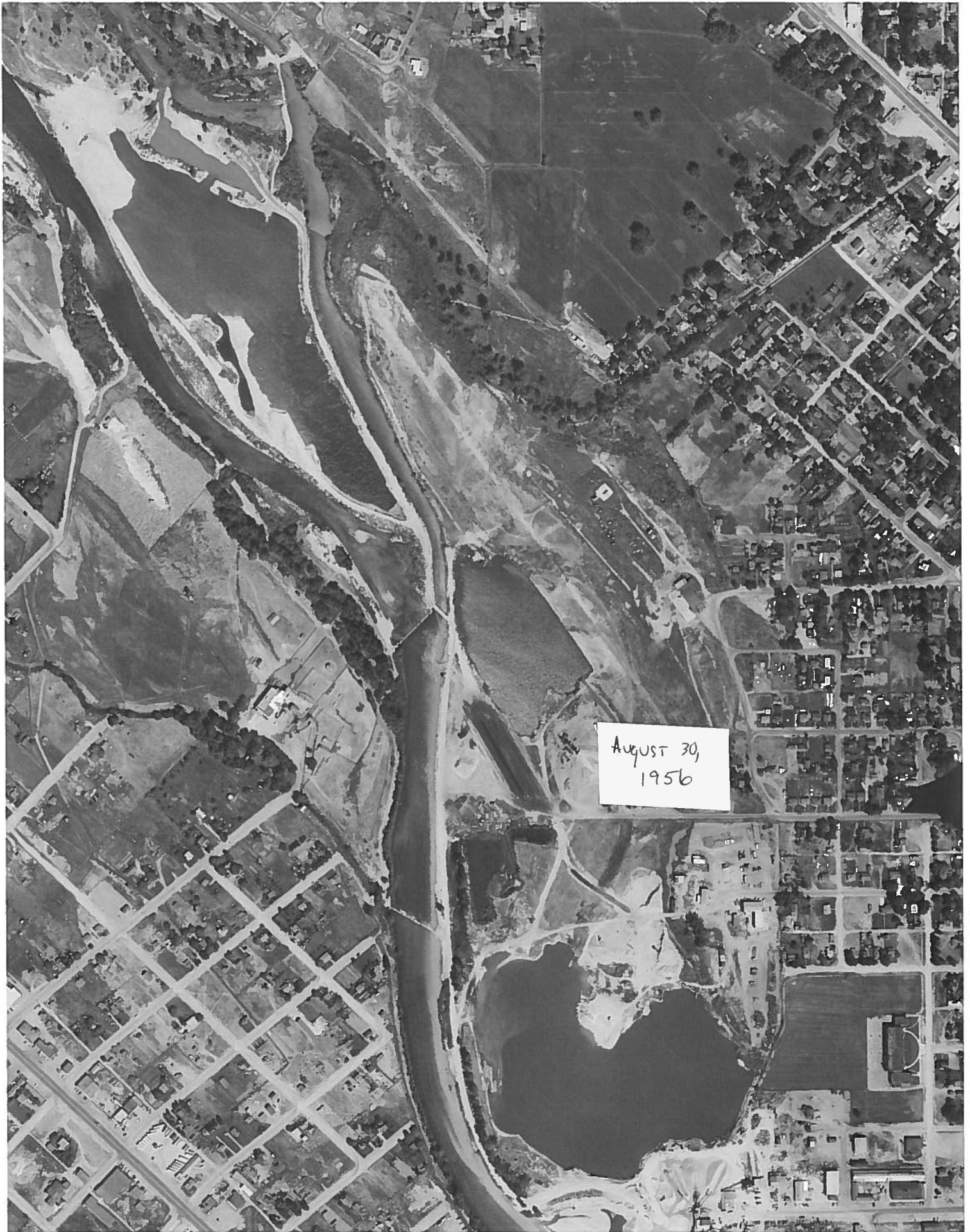
Rego 1 on Grand River - Cross River Dike & Longwood
