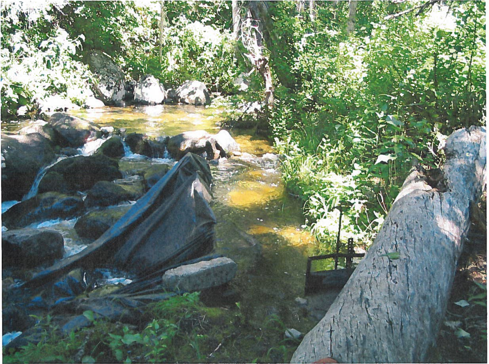
A0014027 Ward or Cunningham Ditch P00 Taken By BOSCO Foster July 21, 04
