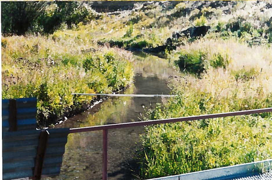
Looking No. over the survey road to the diversion box around the curve of the ditch standing on screen structure 10 35 AM.
