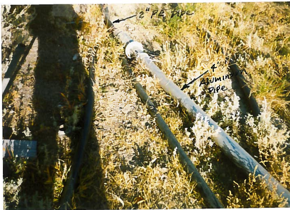
2" polyethylene pipe connected to 4" dia. aluminum Pipe main line.
