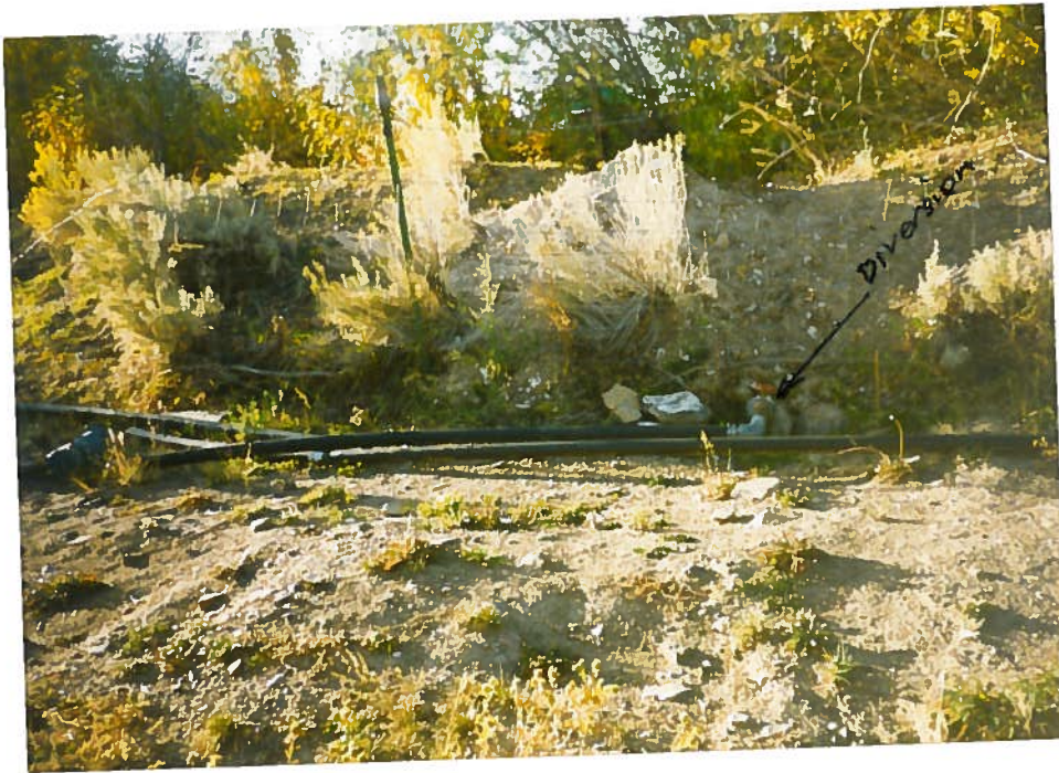
Pipe thru High Line Canal bank supplies the pump
