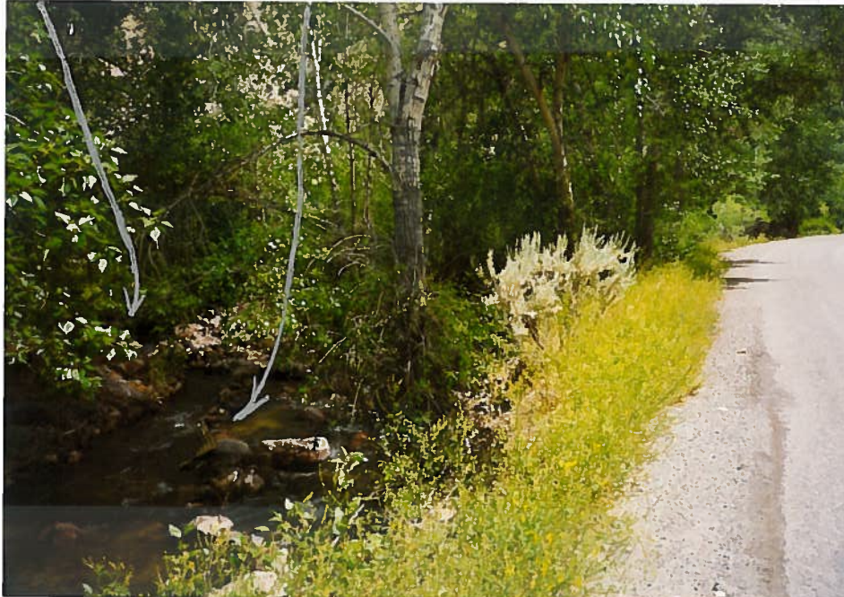
DITCH DIVERSION WORKS
