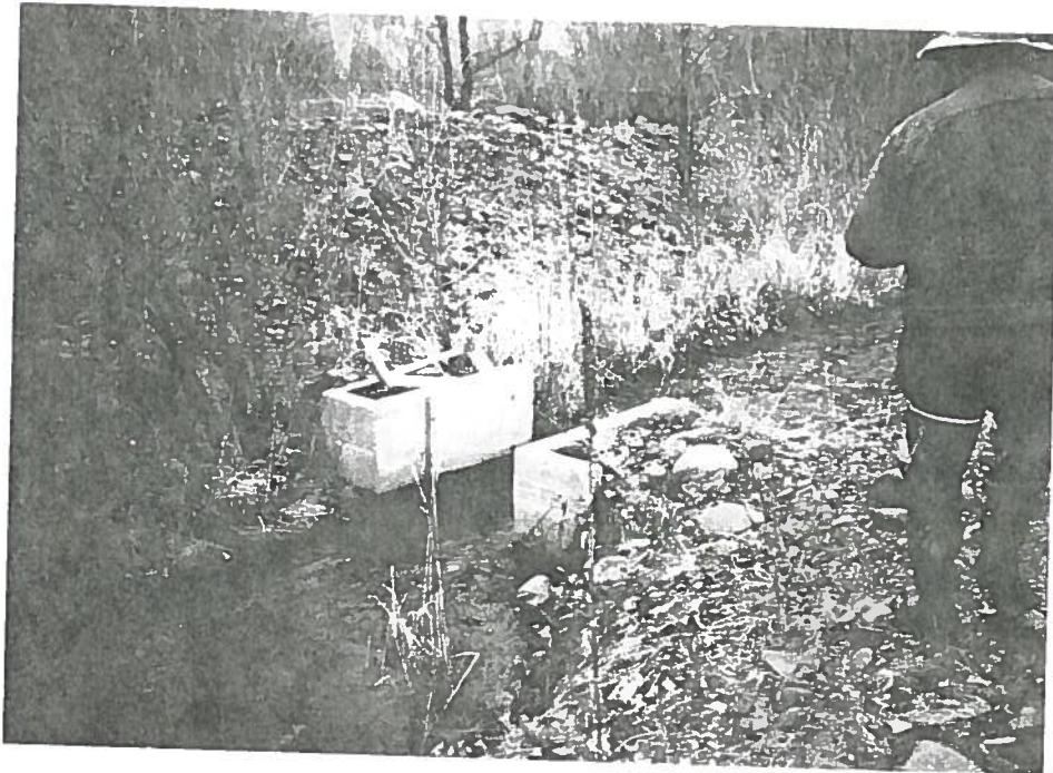
Measuring point for "Bradbury" ditch Note removable wier blade on left side of structure Lester Bradbury at right SENWNE Sec. 8. T14N R19E
