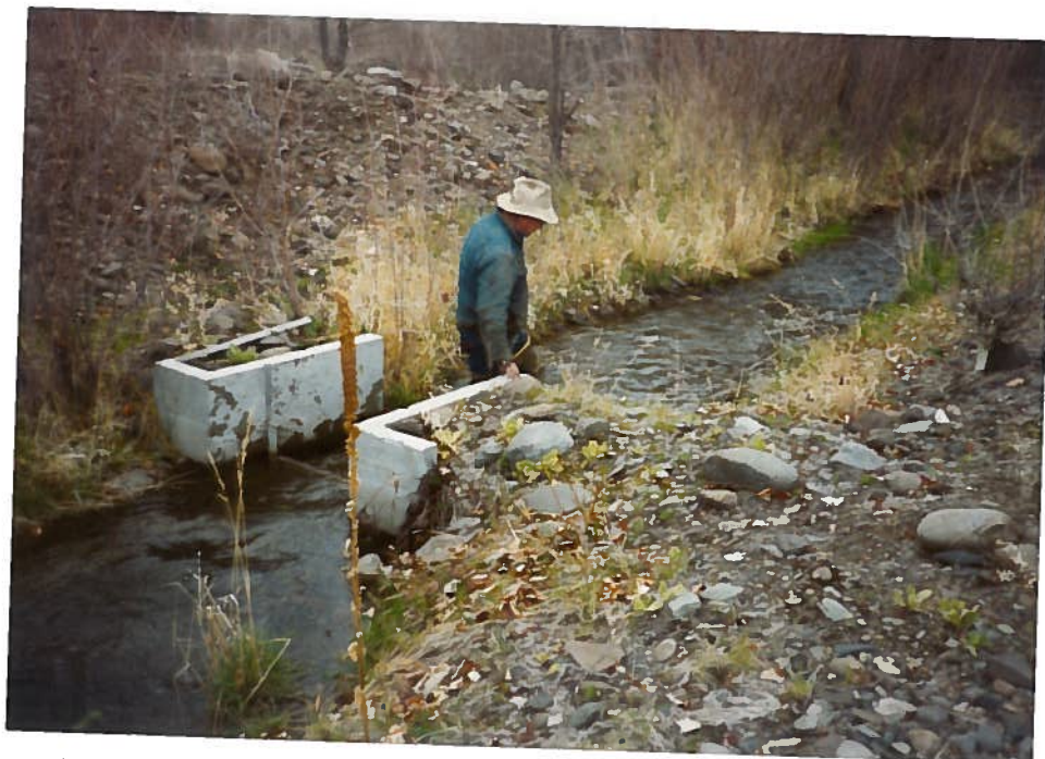
As above Lester has put the removeable blade in place.
