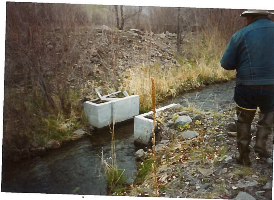
Measuring point for "Bradbury" ditch Note removeable Wier blade on left side of structure Lester Bradbury at right
