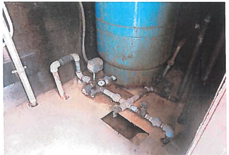
PRESSURE TANK AND COMPONENTS
