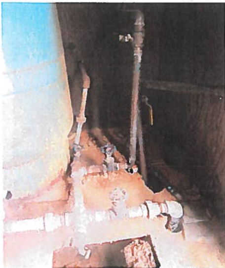
PRESSUSRE SWITCH AND GAUGE
