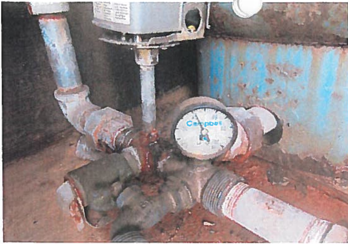
PRESSUSRE SWITCH AND GAUGE
