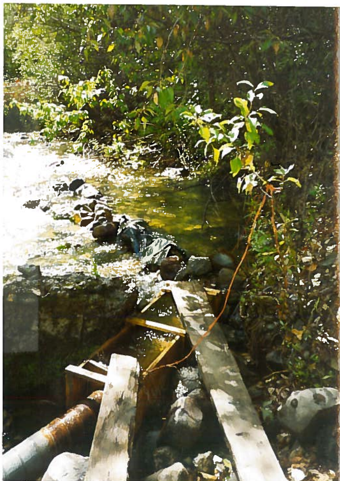
Keefe Diversion point from Mill Creek Diversion box with orifice plate measurement
