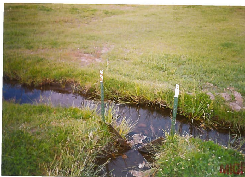
Sullivan's V Notch Weir Measuring Structure
