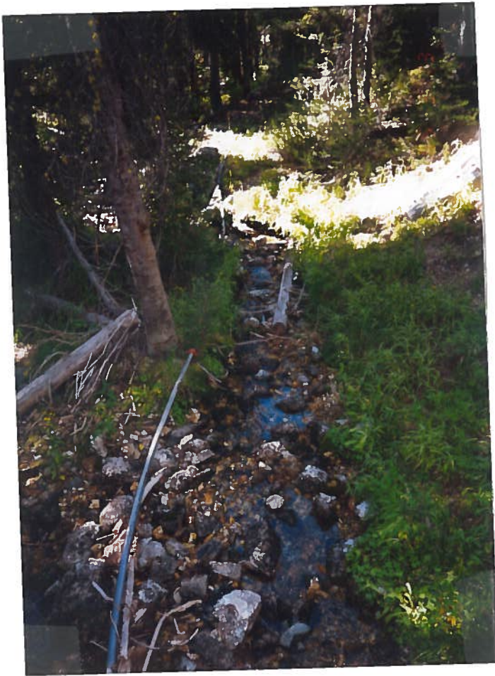
PIPELINE to MINING SITE.
