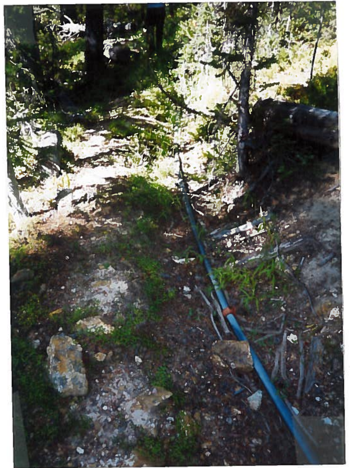
↑ NOTE OLD DITCH BED USED IN PAST MINING OPERATIONS
