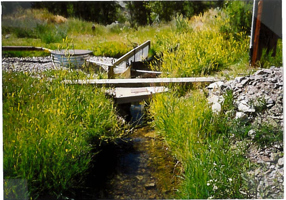
By Pass Ditch AROUND TURNER pump.
