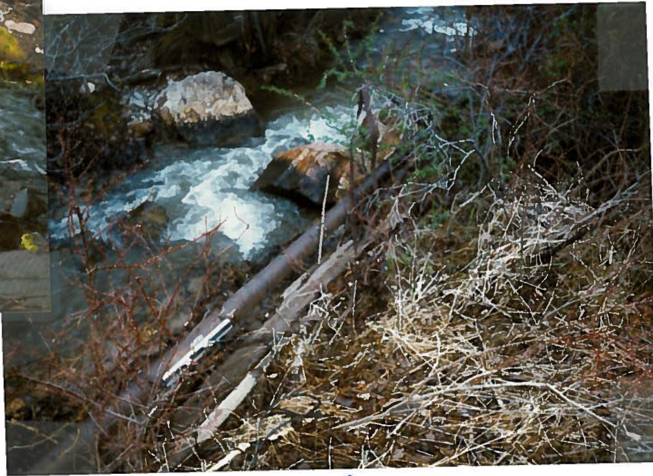
← POLYSONIC METER ON CITY'S PIPELINE.
