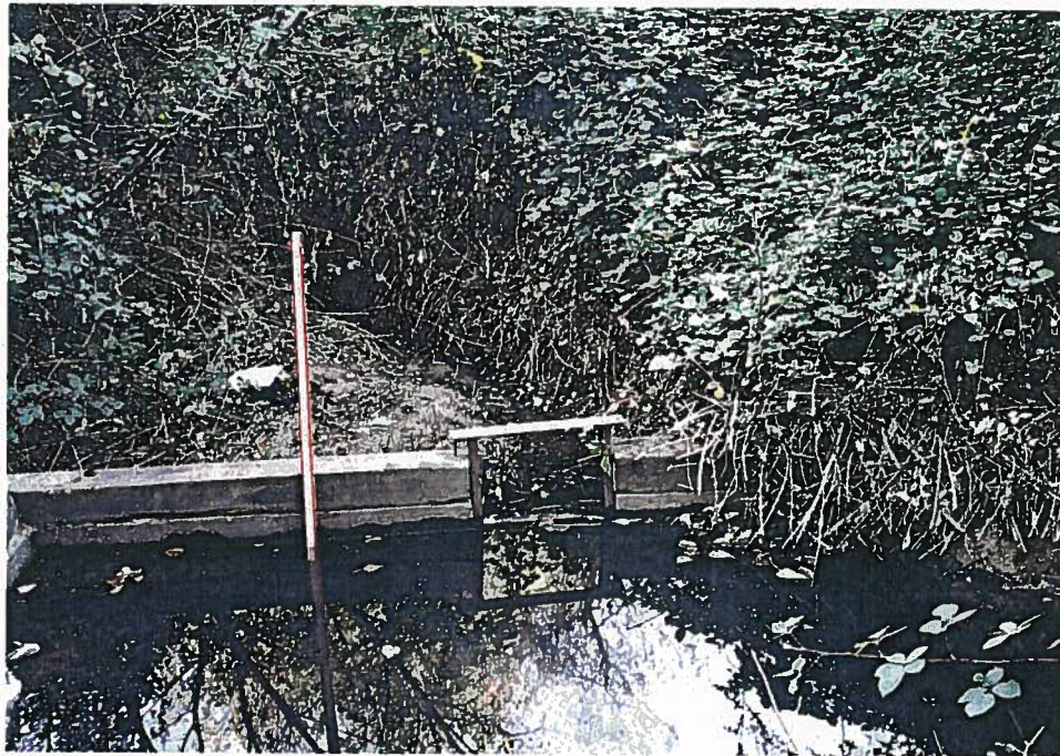
Figure 8. Photographs of the upper impoundment structure for diverting Crane Creek by Crane Creek Country Club golf course. The upper photograph shows Diversion #1 (Upper Weir Diversion) which dams the main channel of Crane Creek. The head gate for CCCC's diversion, on the left side of the photo, is allowing 20 gpm to flow to CCCC's Clubhouse pond in this October 16, 2004 photograph. The lower view shows the impounded creek with CCCC's diversion ditch and head gate in center of photograph. The dimensions and works are described elsewhere in this report
