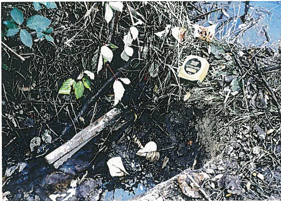
Figure 13. Photographs of the Lower Weir Diversion Ditch and buried control valve. The dimensions and works are described elsewhere in this report and located on Figure 1.
