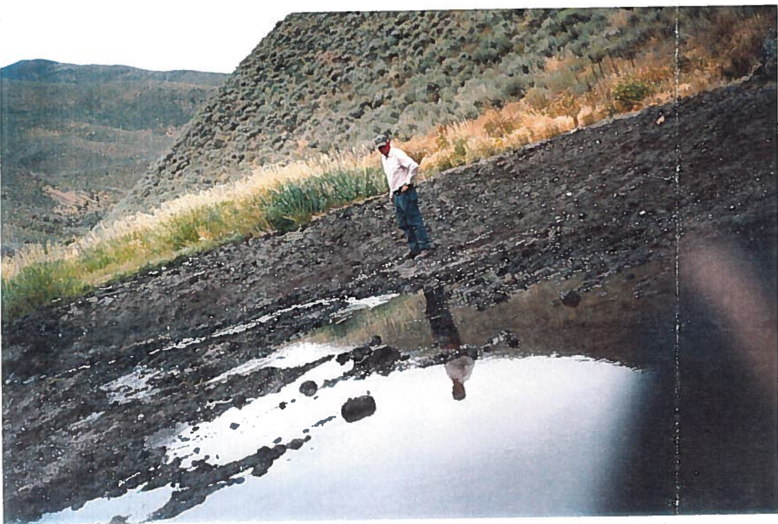
September 9, 2003. Don, looking at water collecting in clay-based soil of excavated pond bed.
