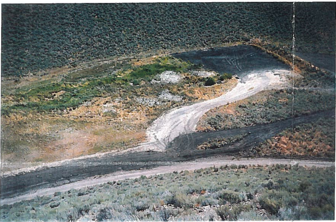
Reservoir/pond after excavation of 3' of silt. One acre of open water. Shows fill used to close old road areas, and new road (2002) just north of RV pad.
