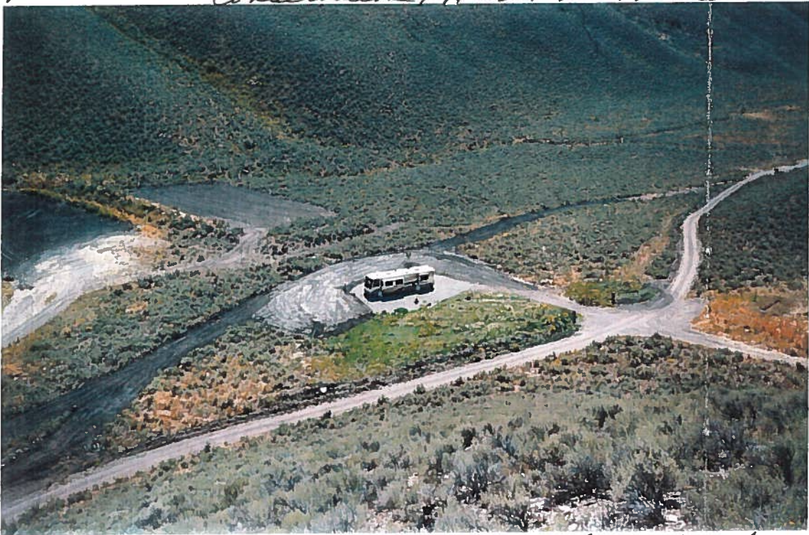
RV pad with new firebreak turning from reservoir/pond silt. New horse pasture area south of dam. Shovel of overflow channel west of dam
