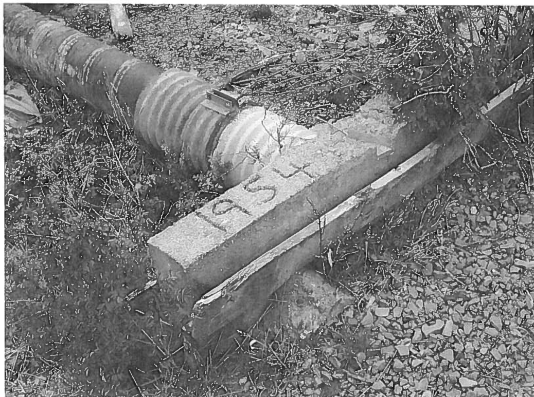
Concrete headwall on outlet works of Copper Creek Reservoir showing date Photo date 10/19/06
