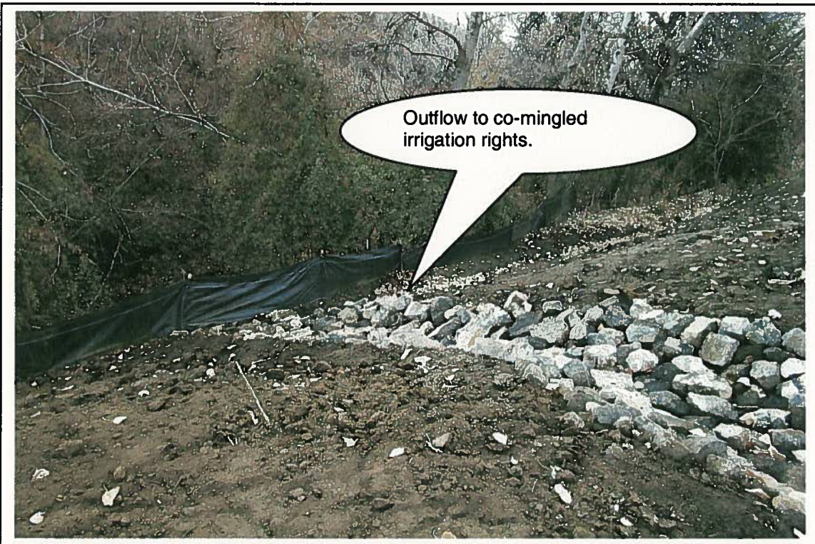
Photo 6: McFarland Creek water right 63-31585 ditch from the pond, which has co-mingled overlapping spring irrigation right 63-31247. Irrigation located in the NWSW, S29, T05N, R02E.
