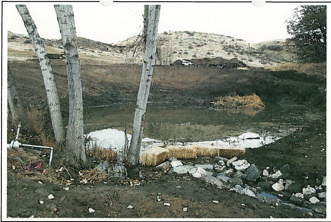
Photo 5: This pond is storage for spring irrigation right 63-31247 and enlargement fire protection right 63-31586. Water is co-mingled. This pond also used as part of the diversion works from McFarland Creek right 63-31585. Pond is too small for storage from McFarland Creek source because it can fill in less than 24 hours with the recommended CFS. The historical McFarland Creek POD to this pond is shown on photo 2, POD 2. Per Matt Howard, Attorney for claimant.
