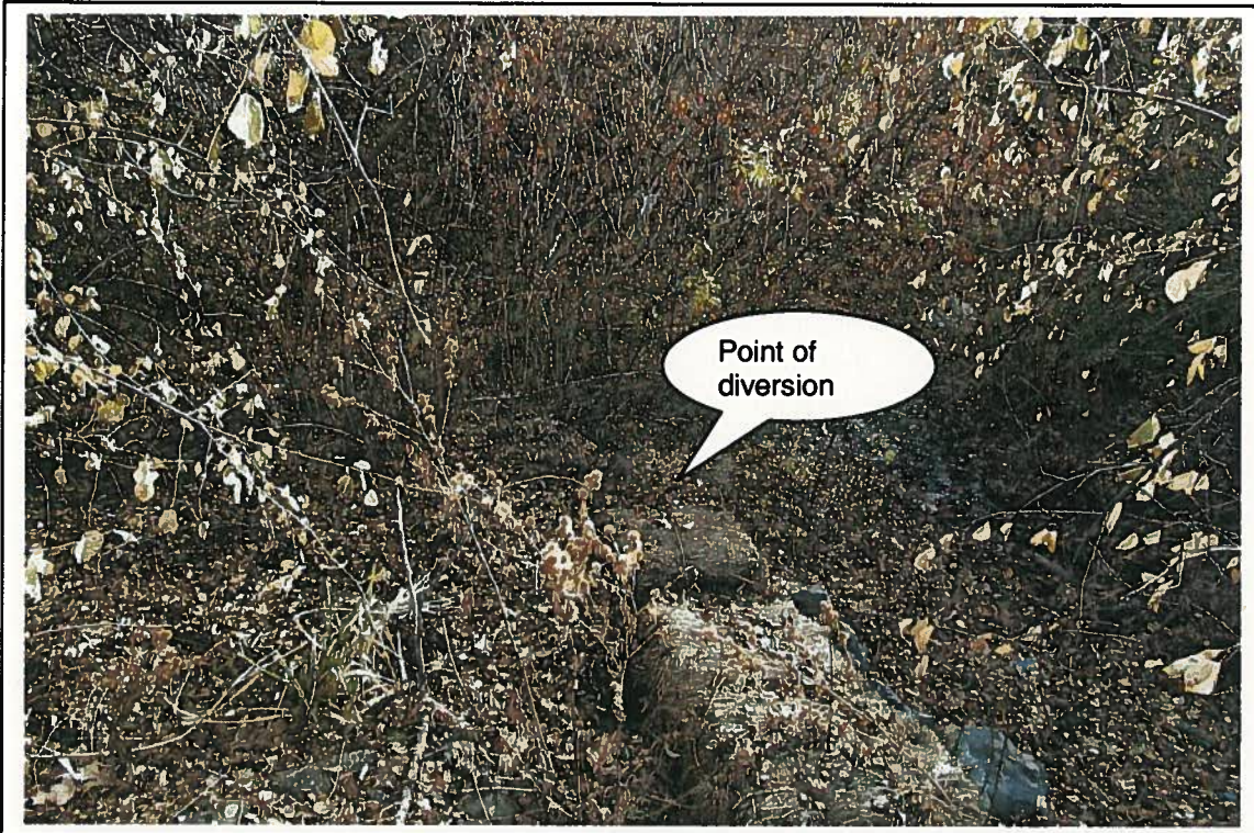
Photo 3: This McFarland Creek POD 3 is located in the NWNWSW, S29, T05N, R02E. This ditch carries both spring and McFarland Creek water. See attached topo layout. Earth rock dam.
