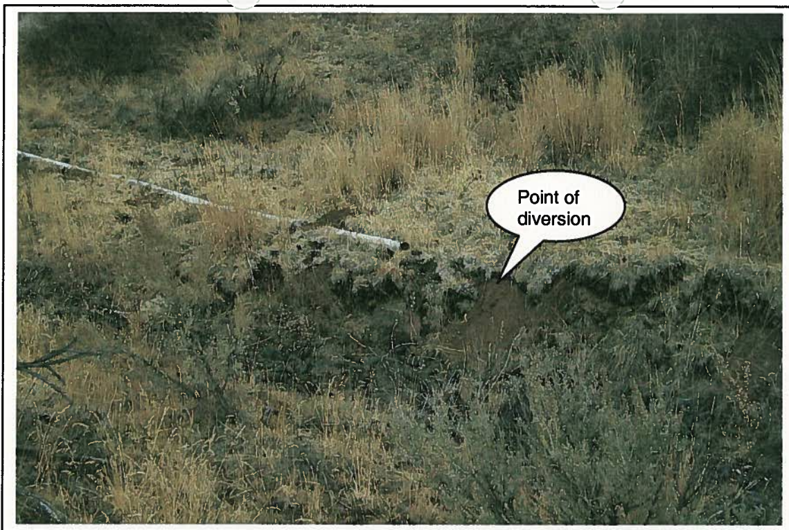
Photo 1: 63-31585, Field Exam 11-15-02: POD1 from McFarland Creek located in the NESW, S29, T05N, R02E. Location shown on 1987 NAPP. Gravity flow ditch. Manning measurement done for this ditch. See 1987 NAPP. Earth rock dam. View downstream.
