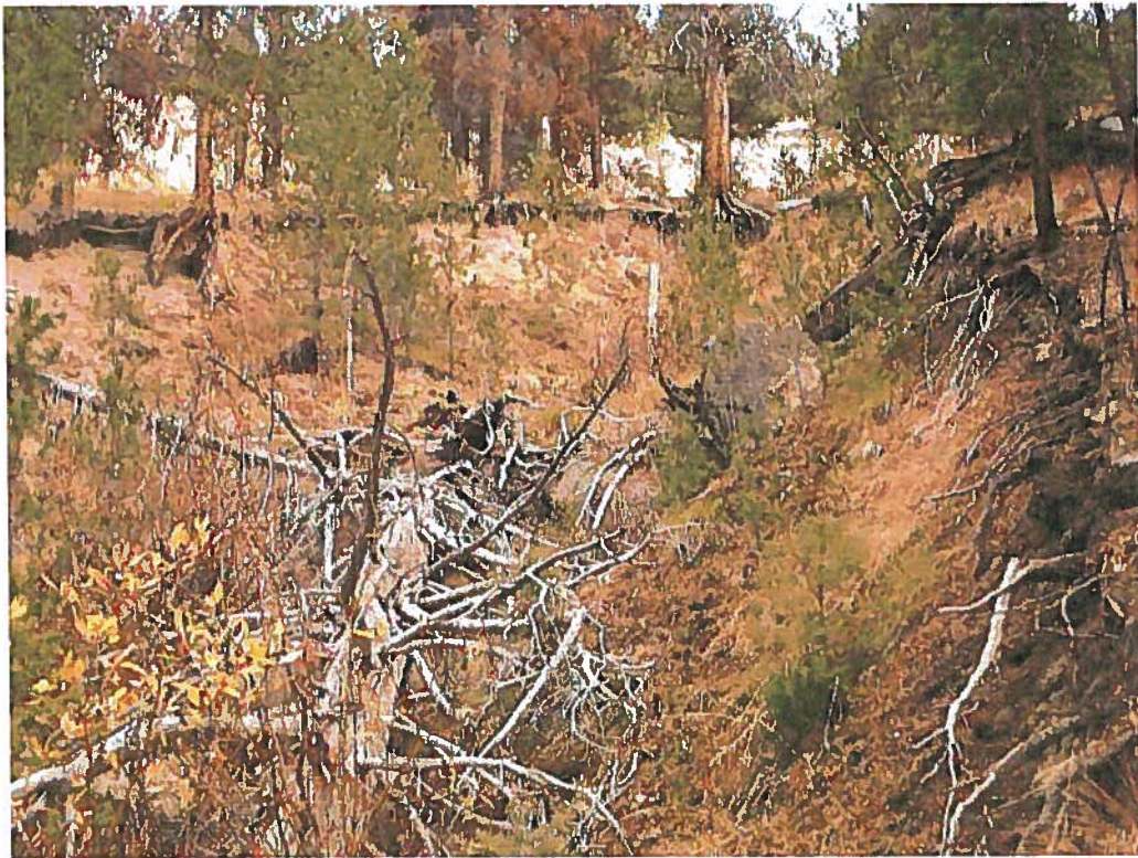
72-2151. Apparent scarring from ditch blow out
