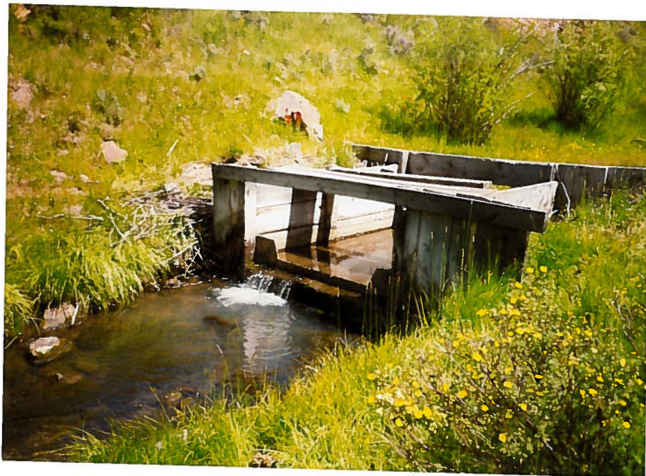
Old Weir Structure - very poor condition
