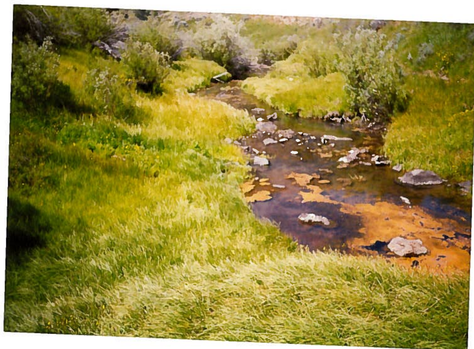
View looking Downstream from outlet Structure. Flow is from seepage thru the dam and some leakage from outlet control.
