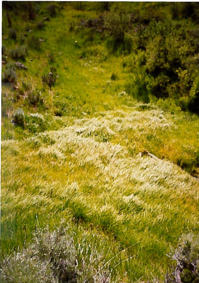
View looking up-slope along the toe of the right embankment.
