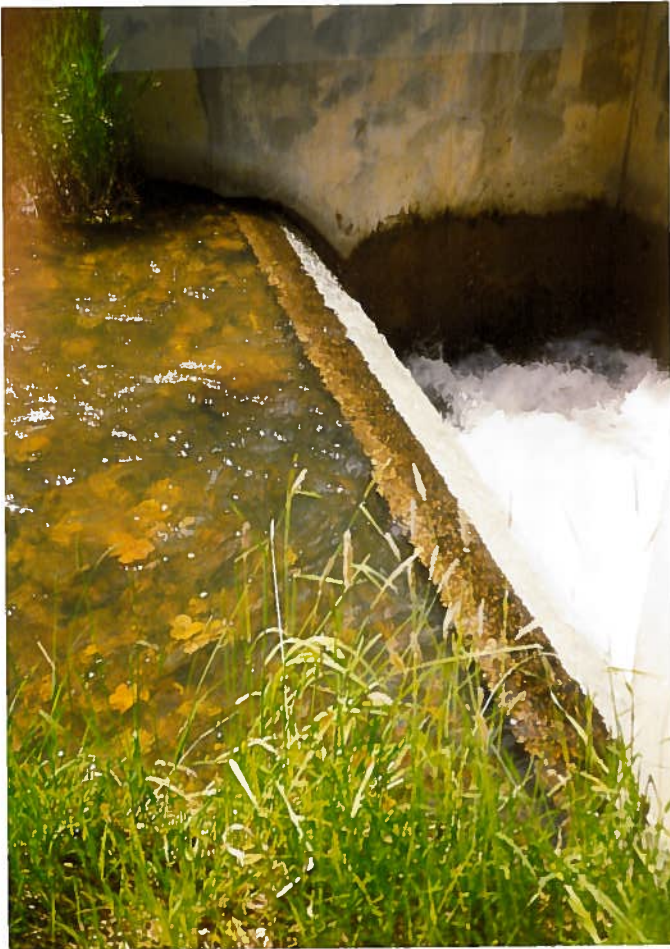
Concrete Sill with overflow at top of Spillway Chute
