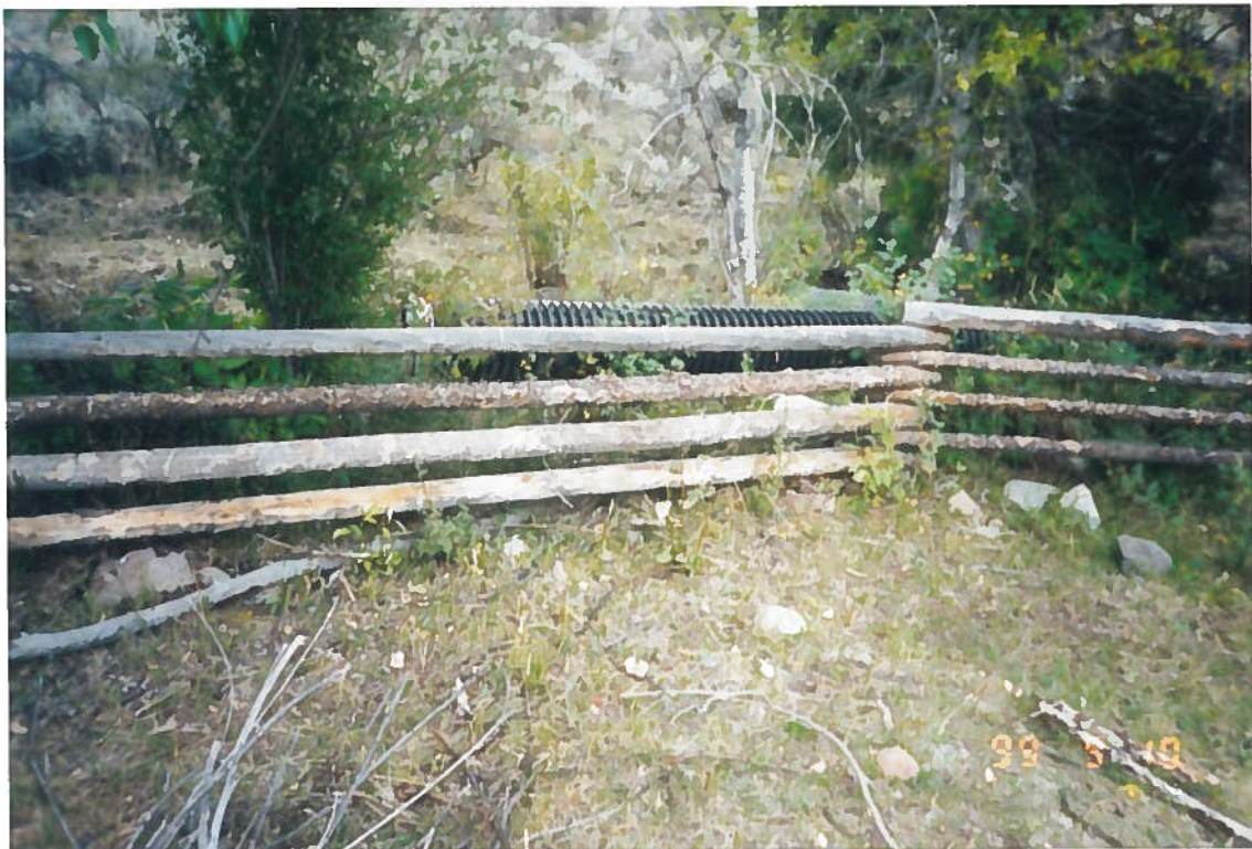
Pipe line being installed to convey Bowery Cr water along E side of property. Photo Taken looking East, just south of Howell House
