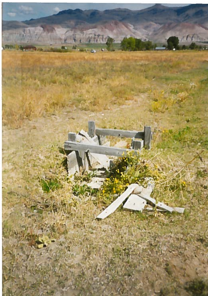
Linda Curtis Claim 72-00032K - Deteriorated Check and Control structure - Near south edge of field in SE \frac{1}{4} SE \frac{1}{4} Sec. 17 View looking East.
