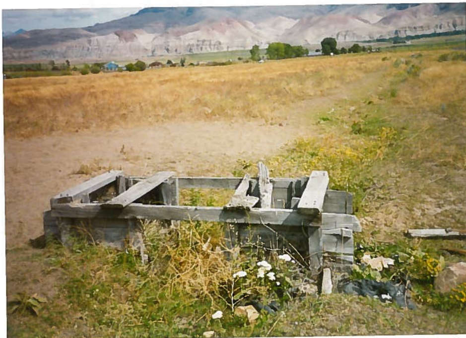
Linda Curtis Claim 72-00032K - Deteriorated Check and Control structure - Near south edge of field in SE \frac{1}{4} SE \frac{1}{4} Sec. 17 View looking East.
