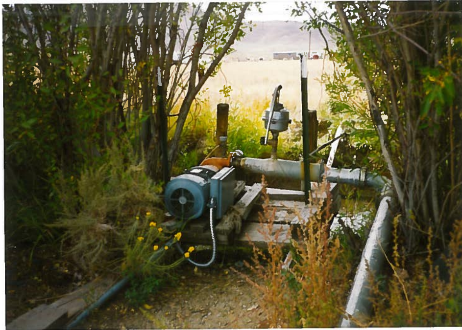
Yacomella Pump Station - Supplies water from the High Line Canal to Sprinklers View looking West
