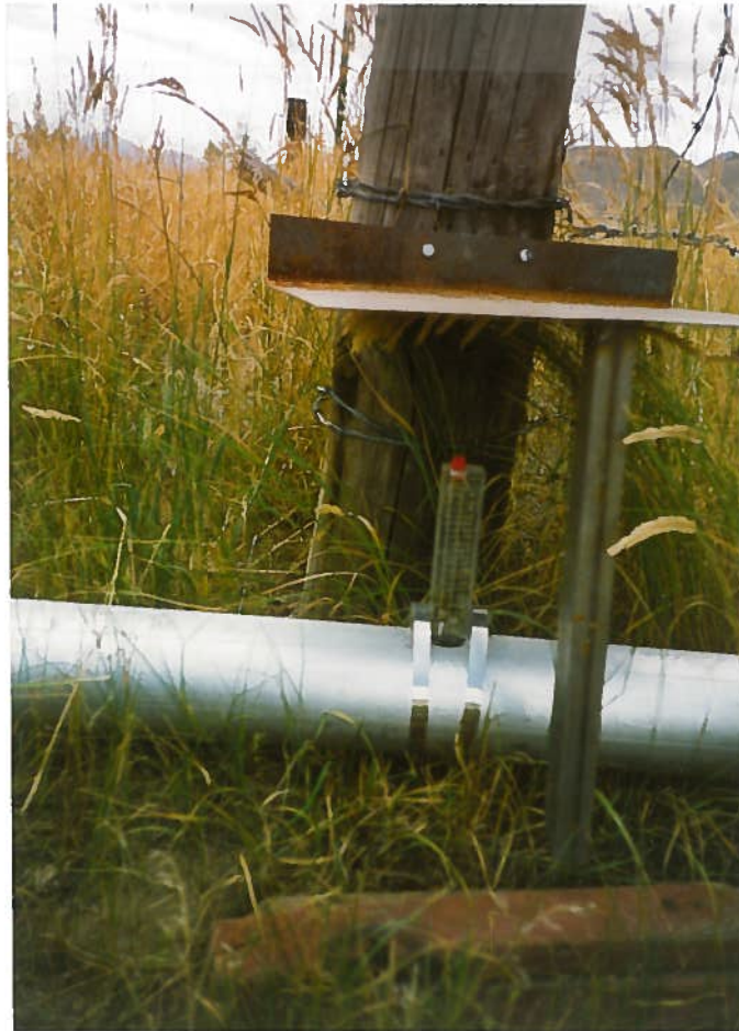
Flow meter on Charles Harvie's 4" mainline Cal Flow Brand - water mark @ 150 gpm.
