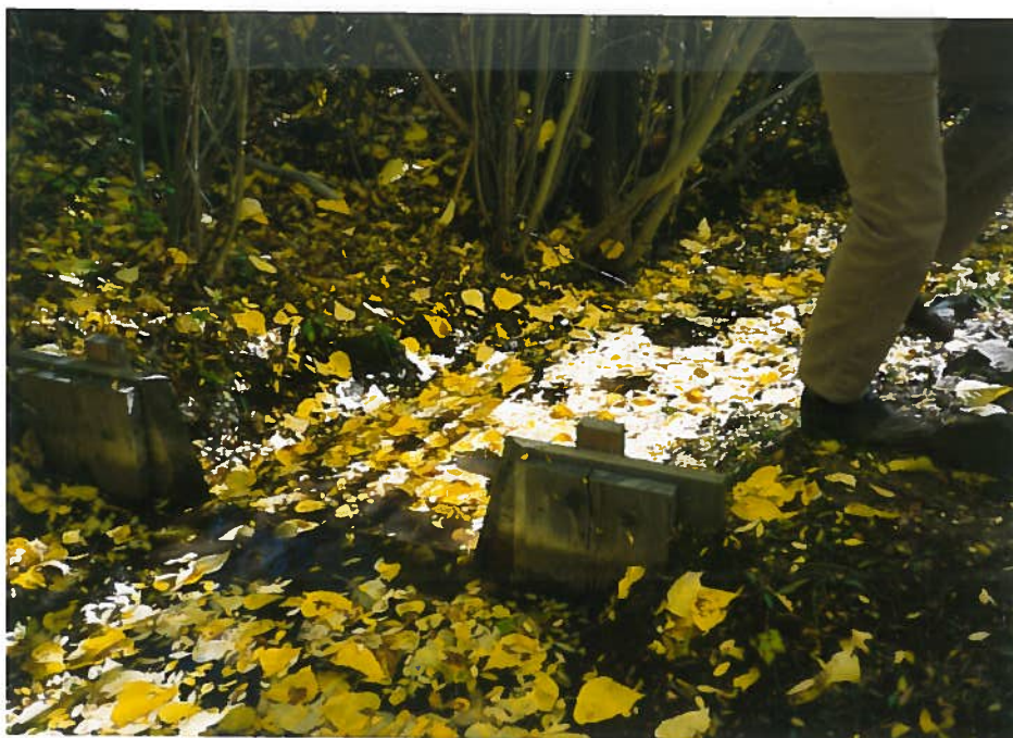
Board weir to measure diversions from Eddy Creek 24" Cipolletti
