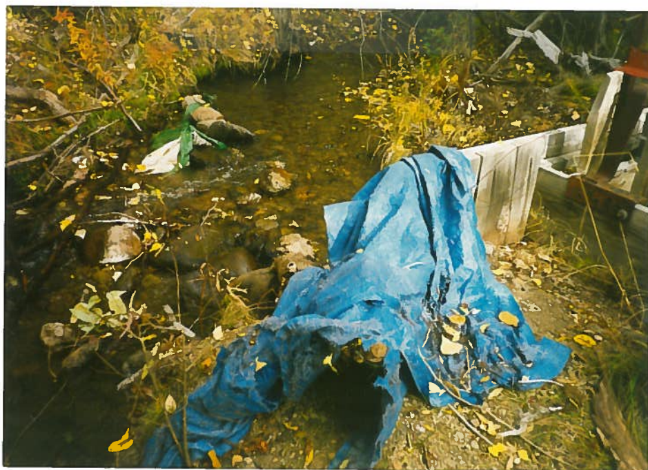
BURCHILL/Raukin Diversion from Eddy Creek Rock Dam with Canvas + wood control gate View looking upstream
