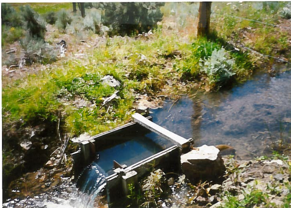
Rankin Weir View looking up stream
