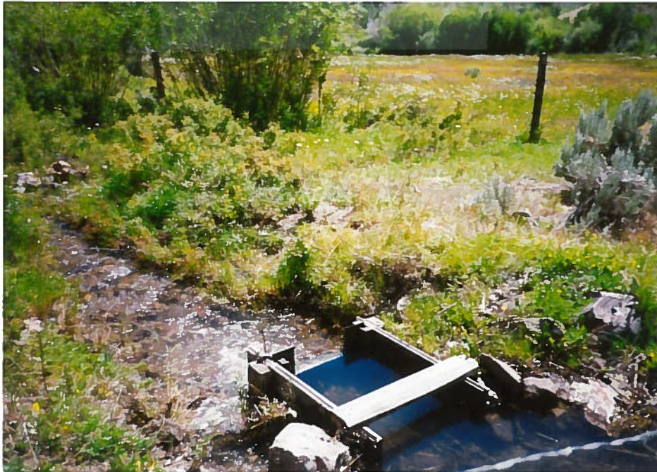
Rankin Weir View Looking Downstream
