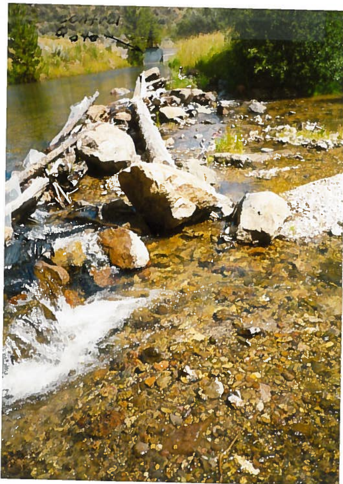
Rock, Log + Plastic check Dam to divert Challis Creek Flow to ditch around the Northwest edge of the irrigated land in Mosquito Flat Valley
