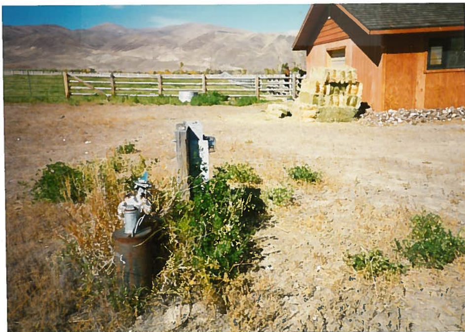
View of groundwater well head with submersible pump. Permit 72-07448.
