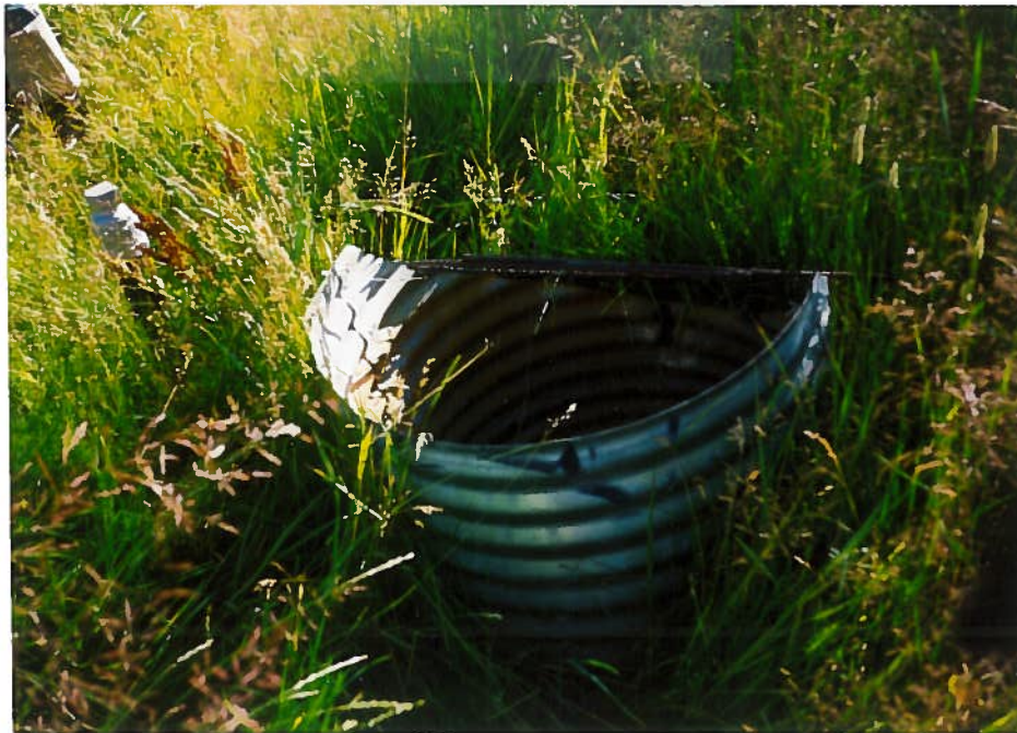
Riser pipe from Artesian well pipeline southward across the irrigated pasture to discharge artesian flows into the conveyance ditch along the south edge of the irrigated pasture.
