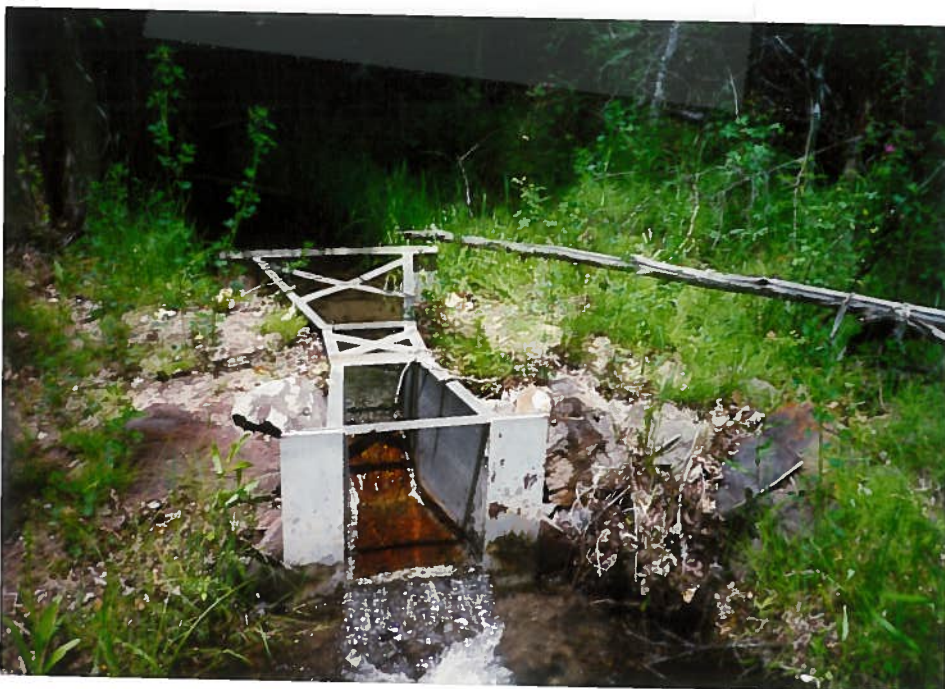
Eddy Creek Parshall Flume - 9" throat
