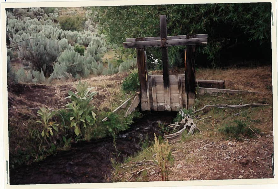
PHOTO #2 REGULATING WOODEN GATE, APPROXIMATELY 10-15 FEET FROM DAM.
