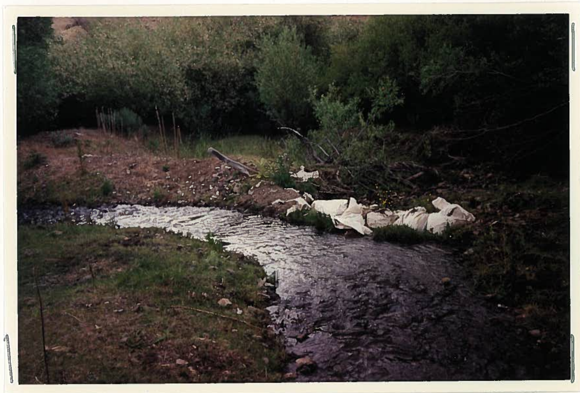
PHOTO #1 P/D, SHOWS EARTH ROCK ETC. DAM IN WILLIAMS CREEK.
