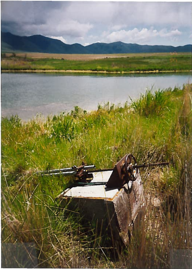
HEADGATE on DAM. View South.
