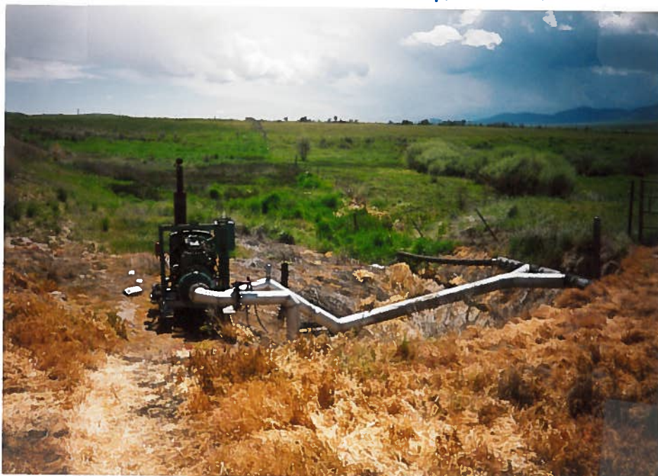
Pump to main line. View South
