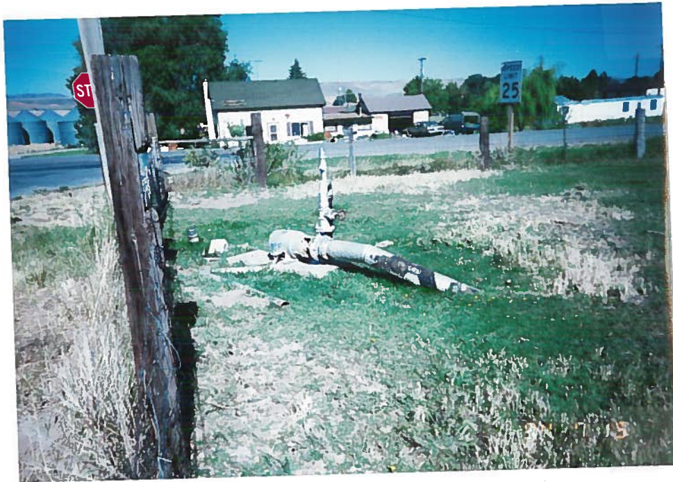
Pump on Rockland Village Ditch To POU Across Hiway.
