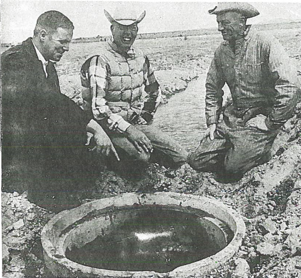
WATCHING water gush from one of seven outlet risers in the new system are D. Ray Guiles, Jim and Ellis Powers. Ellis estimated 50 percent more water now delivered here. Before the new system it took 2½ to 3 hours to
