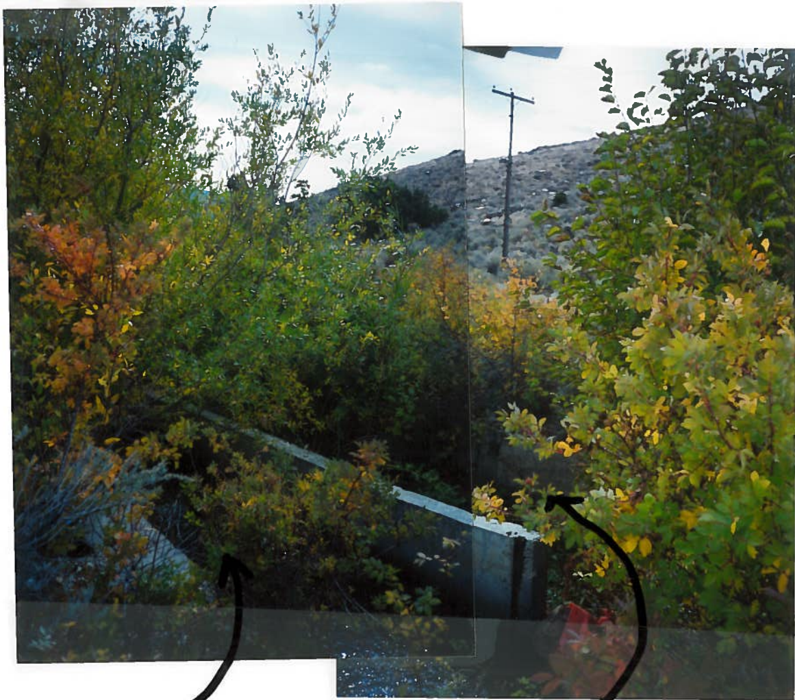
BOWCUT - WICKLE DIVERSION ALSO THE MAIN CHANNEL
