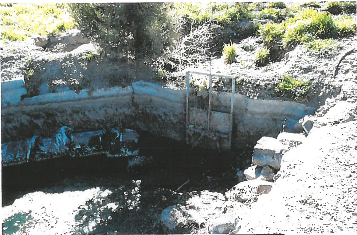
Outlet From Settling Pond To Irrigation Pump By J E Stanton 3-9-05
