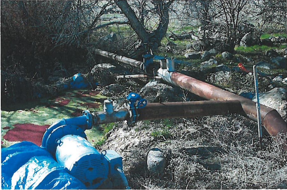
Irrigation Pump, Mainline To Sprinklers – Claim 37-797 By J E Stanton 3-9-05
