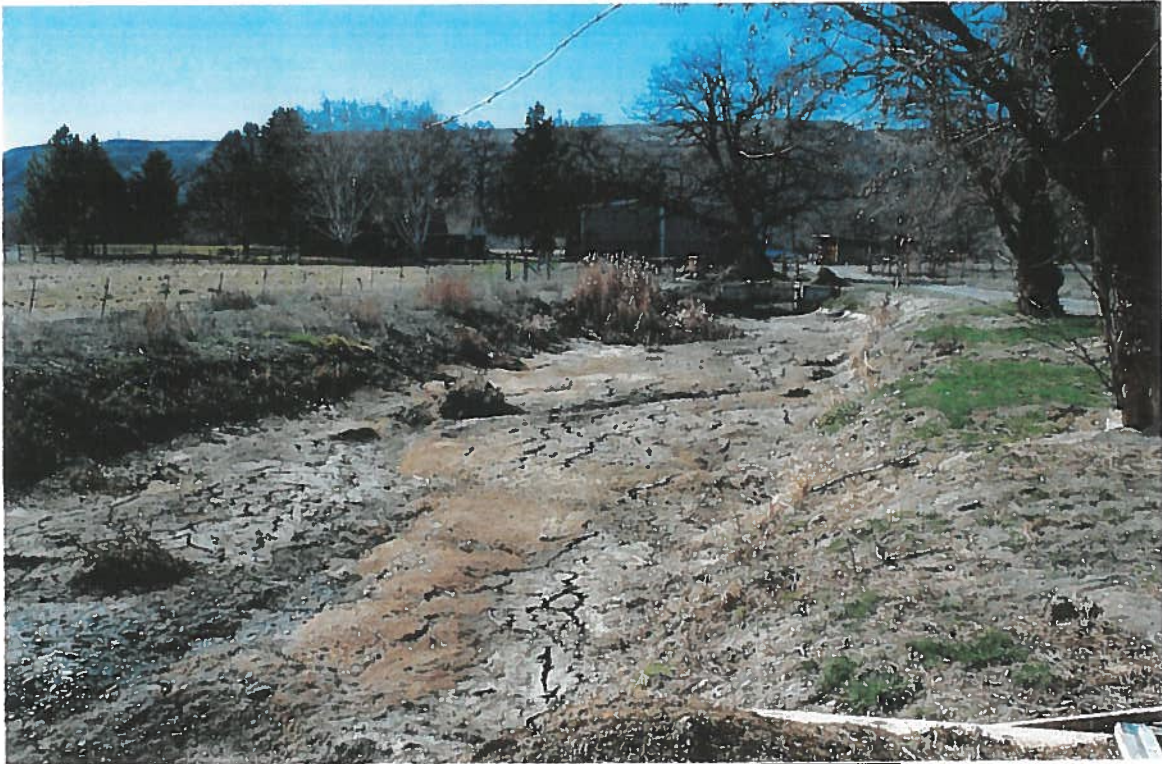
Settling Pond Looking West – Permit 37-7116 By J E Stanton 3-9-05 (Pond dry for cleaning)
