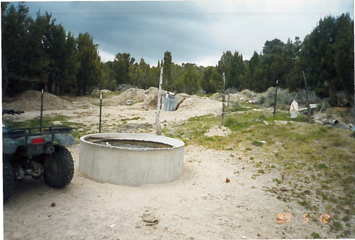
MEASUREMENT SITE #3 Spring fed ditch captured by pipe, conveyed into underground system. Note stock tank in foreground.
