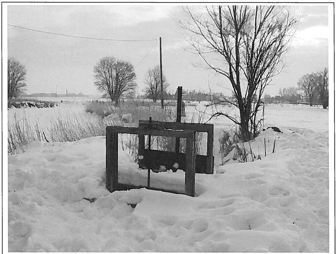
Woodworth Ditch 96 01/28/2004 Tag No. A0011705
