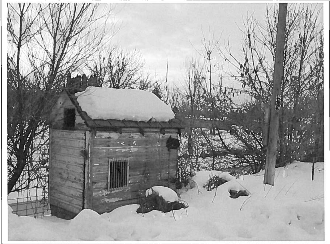
Nevada Street Pump 97-P 01/28/2004 Tag No. A0011708
