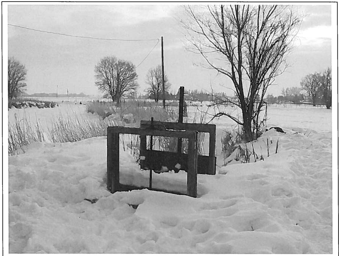
Woodworth Ditch 96 01/28/2004 Tag No. A0011705
