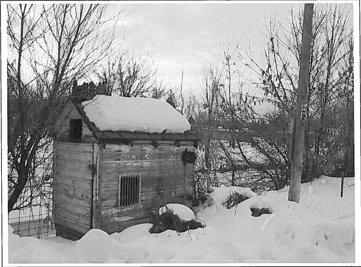
Nevada Street Pump 97-P 01/28/2004 Tag No. A0011708
